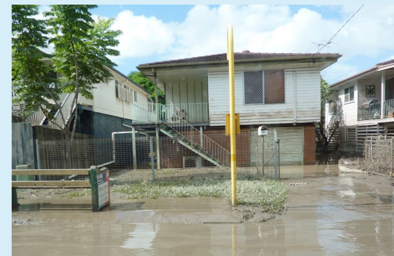
As the waters recede, the tell tale signs of how high up the waters rose still remain on this house at Oxley
